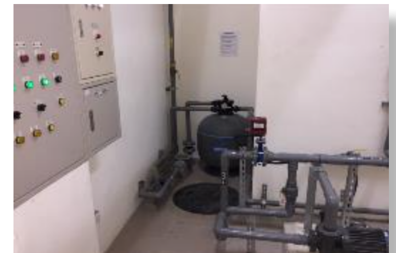
Rainwater harvesting storage system
