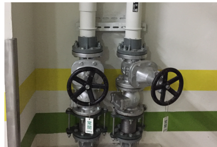
Wastewater treatment: independent pipelines for rainwater
