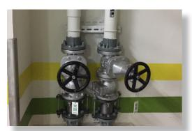
Wastewater treatment: independent pipelines for rainwater
